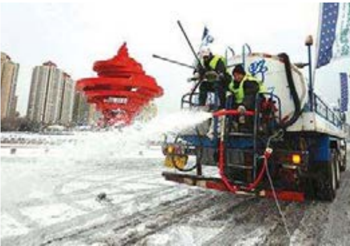
Figure 19 – Spraying snow-melting agents
