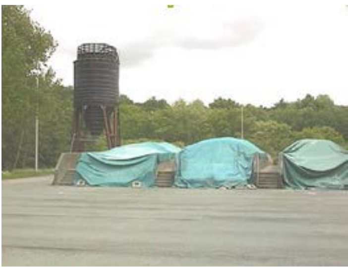
EXAMPLE OF SALT SILOS USED IN BELGIUM
