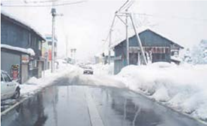
FIGURE 11 - EFFECT OF SNOW-MELTING SPRINKLER SNOW-FLOWING GUTTER
