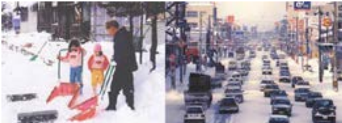
RESIDENTS DUMPING SNOW INTO THE SNOW-FLOWING GUTTER MAINTAINING THE SAME EFFECTIVE ROAD WIDTH IN SUMMER AND WINTER FIGURE 13 - EFFECT OF SNOW-FLOWING GUTTER
